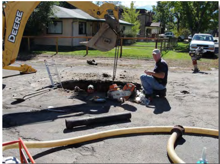
Public Works Repairing Water Lines
