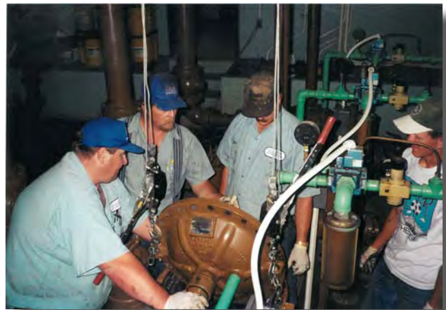
Maintenance and repair of a pump at the Wastewater Treatment Plant
