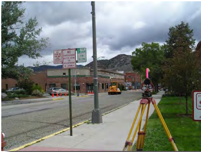
Chip seal project F Street
