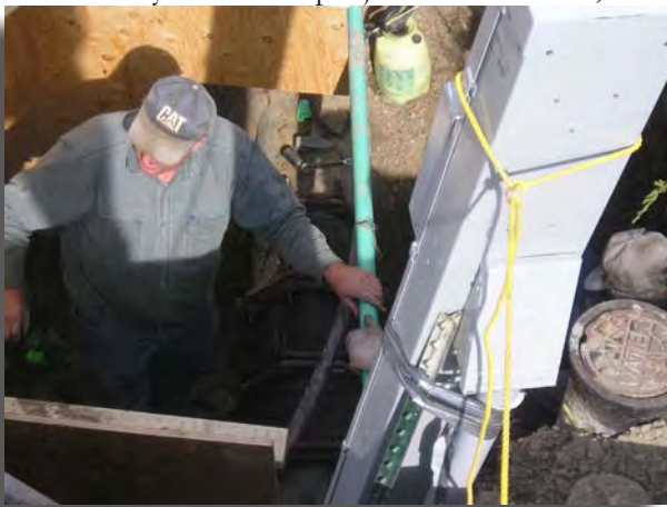
Public Works performing maintenance of city water lines
