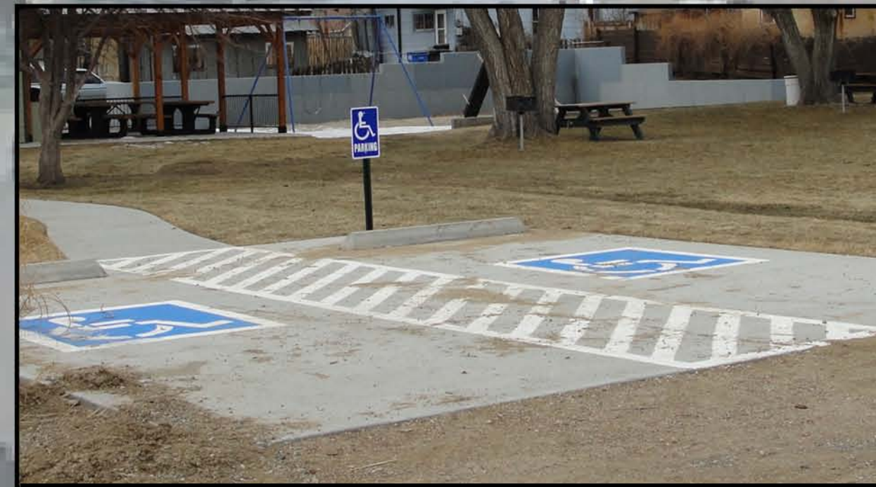
2 New Concrete ADA Parking Spaces
